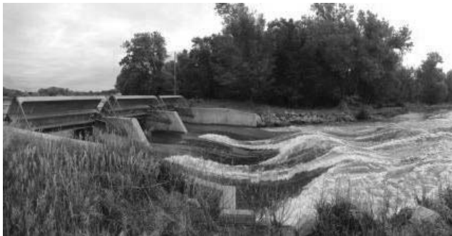
30-Mile Canal Headworks, June 2015
