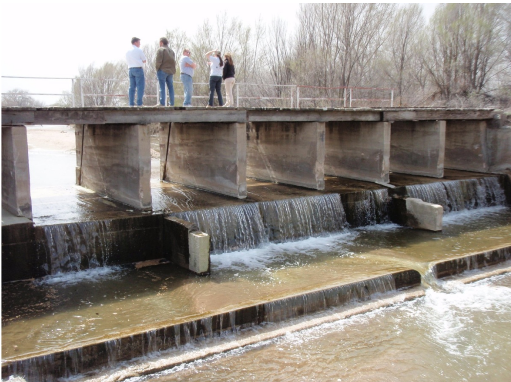
Photo 34 – Downstream Face of Headgates
