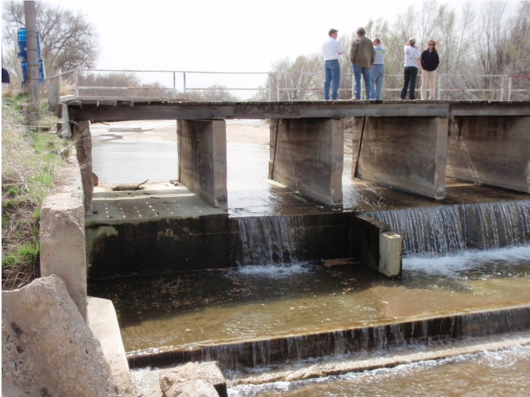
Photo 33 – Downstream Face of Headgates
