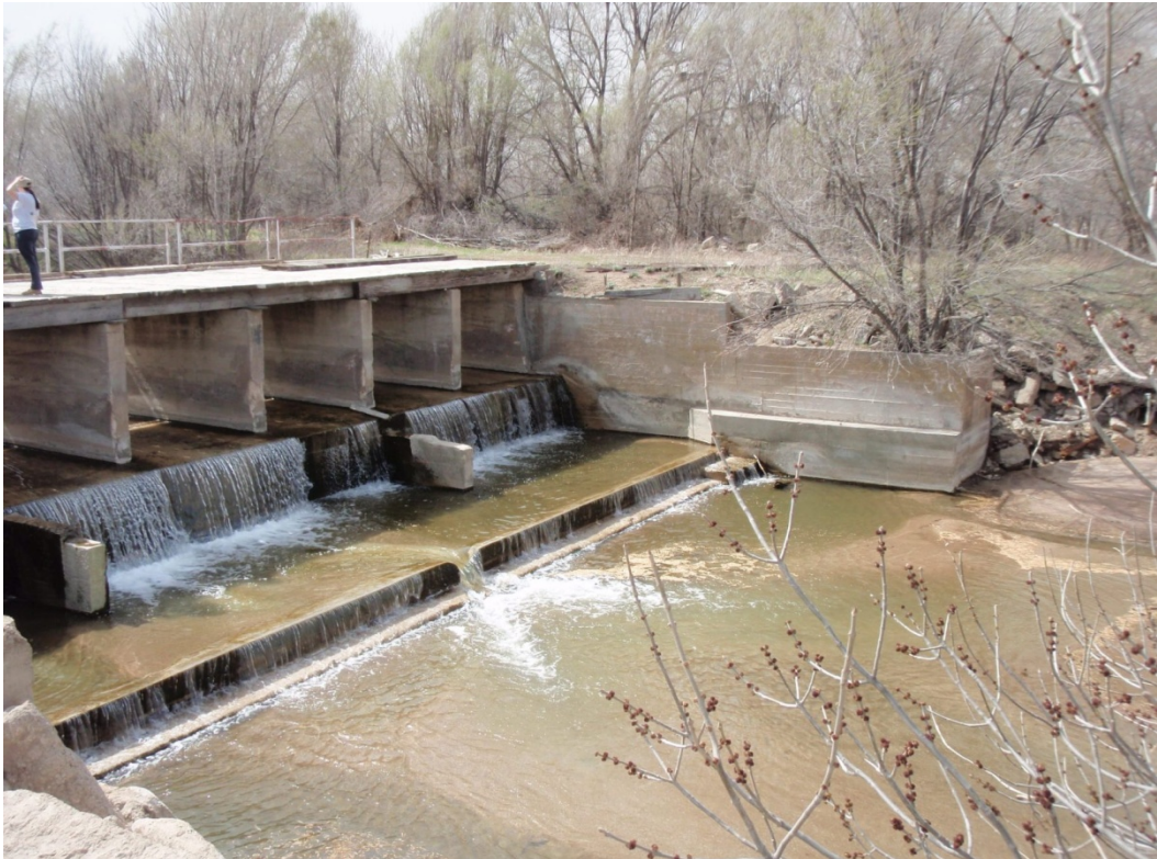
Photo 32 – Downstream Face of Headgates
