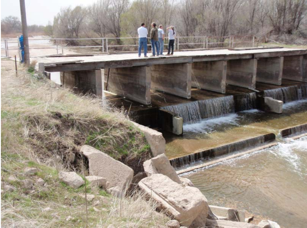
Photo 31 – Downstream Face of Headgates
