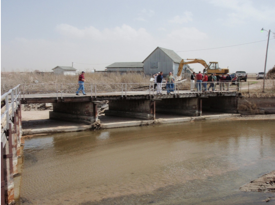
Photo 27 – Upstream Face of Western Canal Intake Structure
