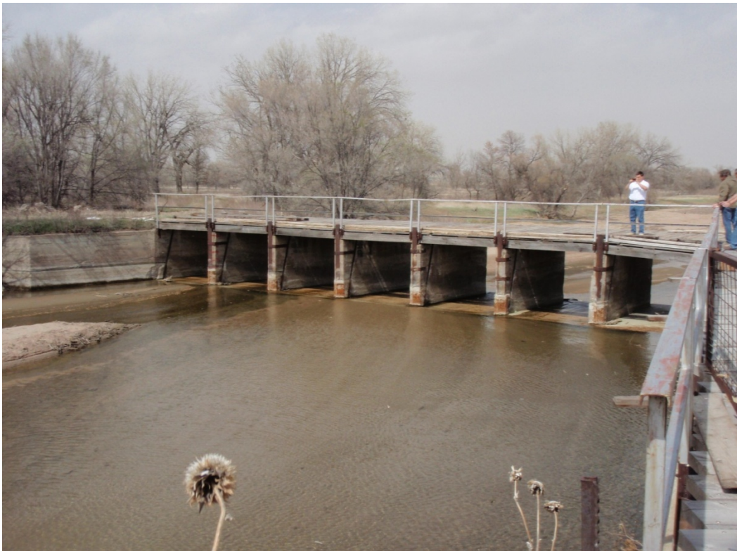
Photo 24 – Upstream Face of South Platte River Headgates
