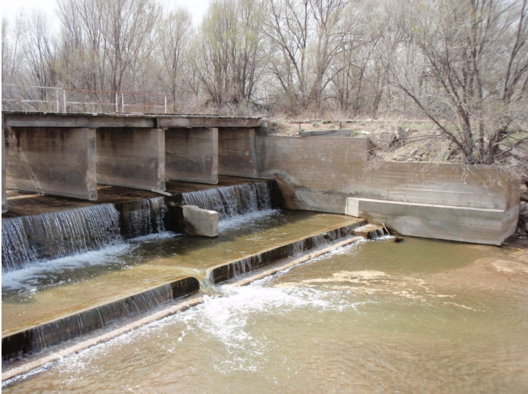
Photo 35 – Downstream Face of Headgates
