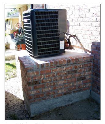
Figure 3-1. Air conditioning compressor elevated on a pedestal.
