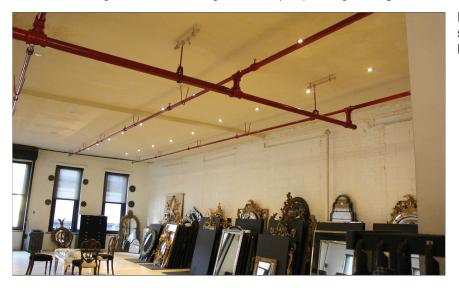
Figure 5-20. Fire protection piping and sprinkler heads installed along the building ceiling.
