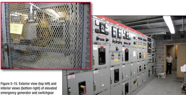
Figure 5-15. Exterior view (top left) and interior views (bottom right) of elevated emergency generator and switchgear at medical center in Galveston, TX. Figure 5-14 is an exterior view of the electric room.
