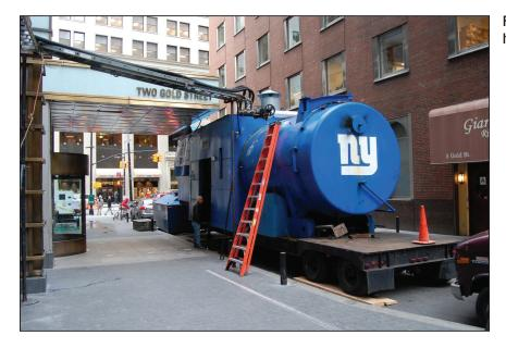
Figure 3-7. Portable boiler provides heat during repair of flood damage.
