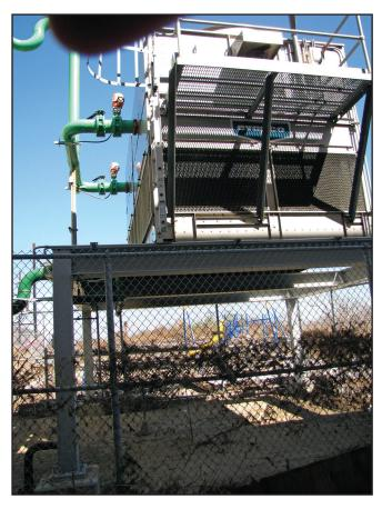
Figure 5-7. Cooling tower placed on an elevated frame (Hurricane Ike, Port Bolivar, Texas, October 18, 2008).
