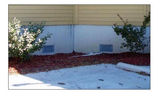
Figure 6-43. Example of flood vents
