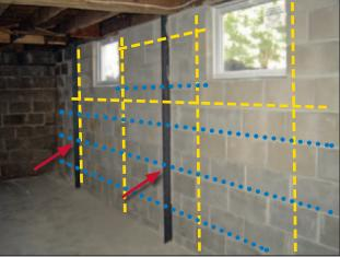
Figure 5D-16. This house's foundation was rebuilt after collapse from saturated soil forces after a flood. The blue lines on the wall indicate locations of internal wall joint reinforcing, the yellow lines indicate location of vertical reinforcing bars, and the exterior reinforcement can be seen in the pictures (red arrows).
