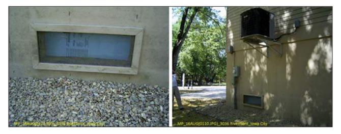
Figure 5E-14. A house where flood openings have been covered by insulation and drywall
