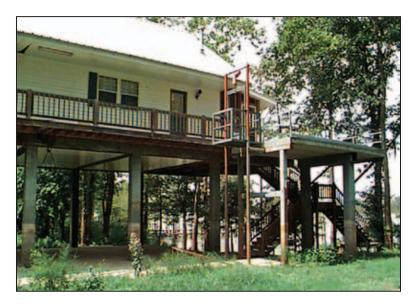
Figure 6-28. House elevated on timber piles
