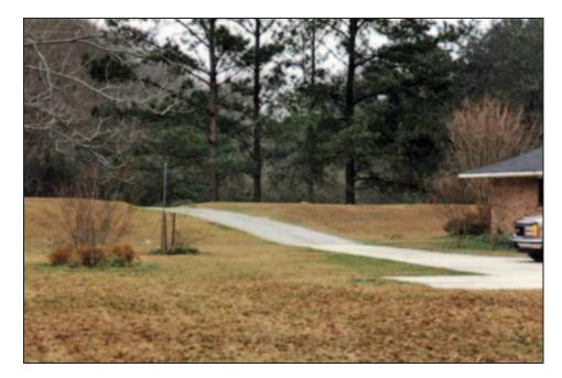
Figure 6-57. Driveway access over a residential levee
