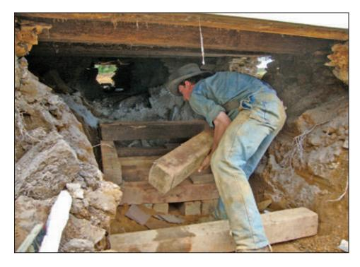
**Install Beams:** Lifting and lateral beams are placed beneath the structure at all critical lift points and support cribbing is added as the structure is separated from its old foundation (see Figure 5R-6).
