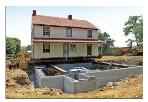
Figure 5R-10. New foundation wall construction begins (photo courtesy of Wolfe House Movers)
