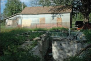
Figures 5D-11 and 5D-12. This house located in the SFHA was displaced from its foundation into the roadway adjacent to it. The photo on the right shows the house's original location.
