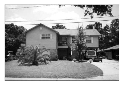
Figure 6-17. Elevation of an existing home above the BFE
