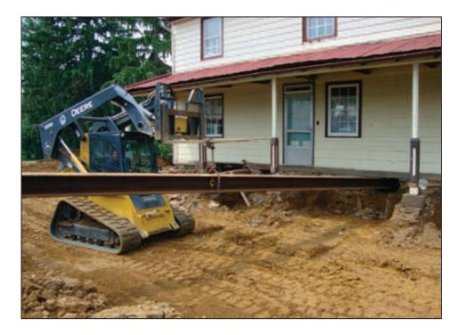
**Install Jacks:** Jacks are used to lift the structure from its foundation (see Figure 5R-7). Various types of jacking systems may be employed as long as gradual and uniform lifting pressures are utilized to lift the structure.
