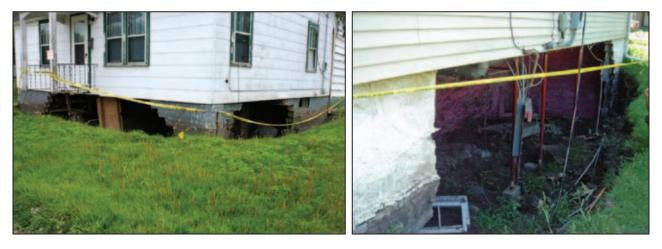
Figure 5D-14. This house's foundation walls were not able to withstand the forces applied during or after the flood. Rebar would need to be added to help with reinforcement of the CMU foundation.
