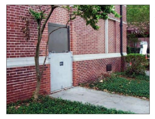
Figure 6-40. Example of a flood shield over a door
