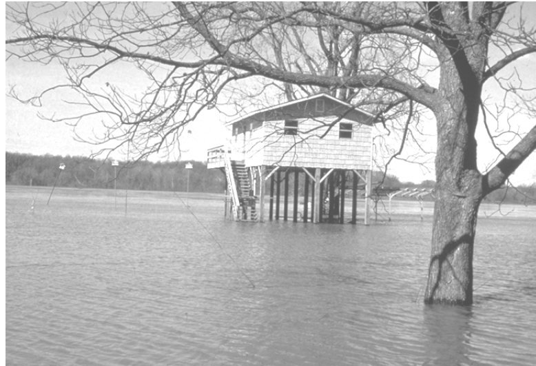
Figure 5-8. Elevation on piers
