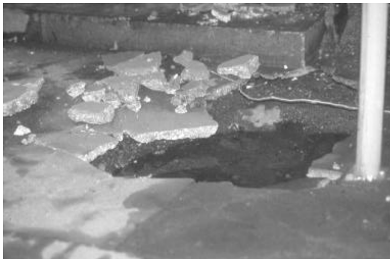
Figure 1-19. This basement floor broke from hydrostatic pressure
