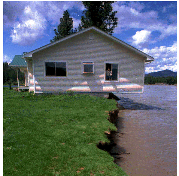
Figure 1-5. Riverine erosion can undercut structures
