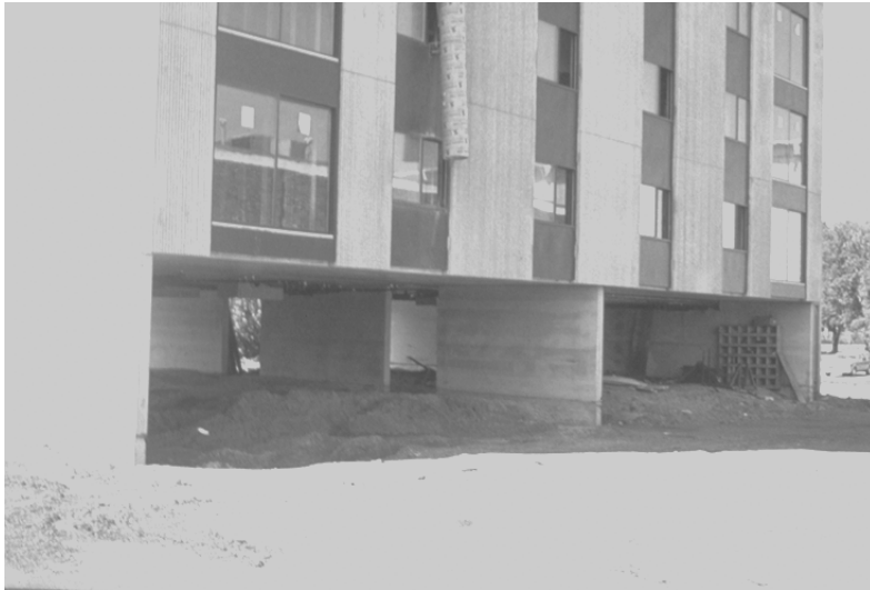
Figure 5-9: Building elevated on parallel stem walls.
