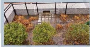
Planter boxes have vertical walls and open or closed bottoms. They are well-suited to collect and absorb runoff in dense urban areas where limited space is available.
