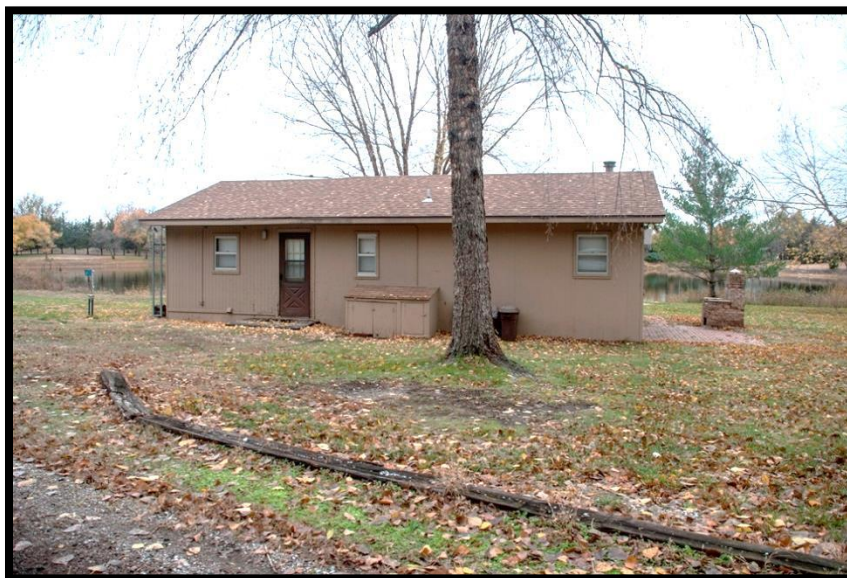
Figure 2. Homes like this one in Cedar Creek have their first floor 4 or 5 feet below the base flood elevation. Elevating this home would reduce flood risk, reduce flood insurance, and make the family safer.
