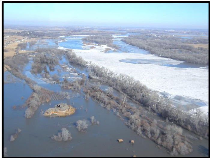
Figure 3. Flooding near Yutan, Highway 92 bridge visible near top of photo. Photo by Papio NRD.
