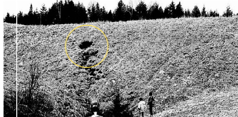
Internal erosion that was discovered in time for the owner to draw down the reservoir and prevent failure of the dam.
