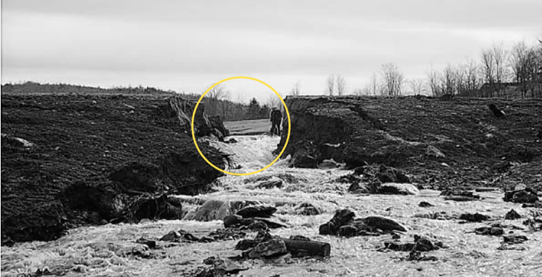
...and later the dam failed!
