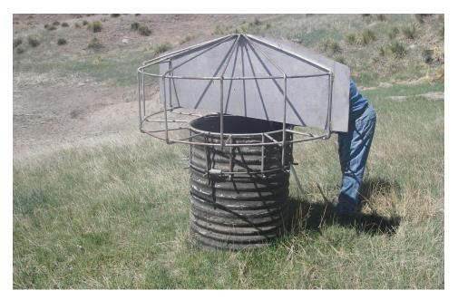
Example of an approved conical trash rack for vertical corrugated metal pipe risers.
