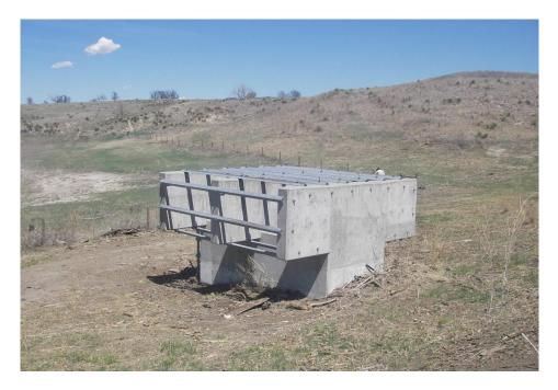
Example of approved trash rack for large reinforced concrete intake structure.
