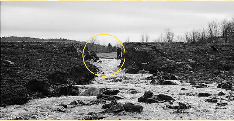
...and later the dam failed!
