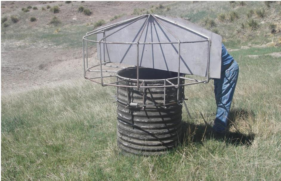
Example of an approved conical trash rack for vertical corrugated metal pipe risers.
