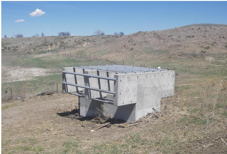
Example of approved trash rack for large reinforced concrete intake structure.
