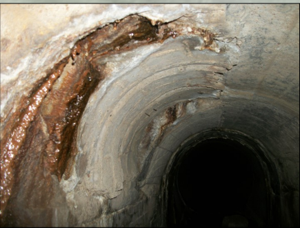
The inside of the Oliver Dam spillway conduit after it was lined in 2019 with a cast-in-place pipe (Photo Courtesy of Miller & Associates and FYRA).
