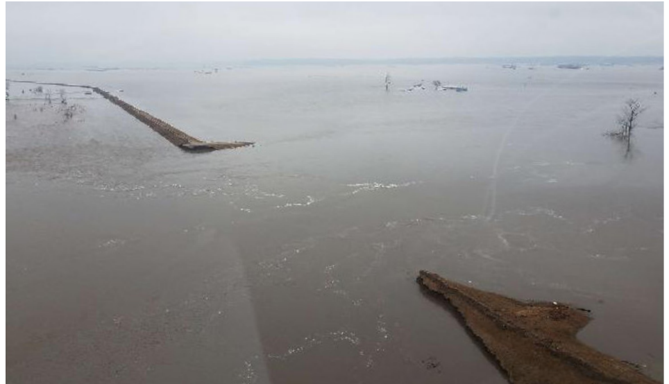
Levee breaches along the Missouri River, like the one pictured above at L-575 near Hamburg, IA, caused extensive damage to property and critical infrastructure such as Interstate-29. Photo taken March 2019, U.S. Army Corps of Engineers Omaha District.
