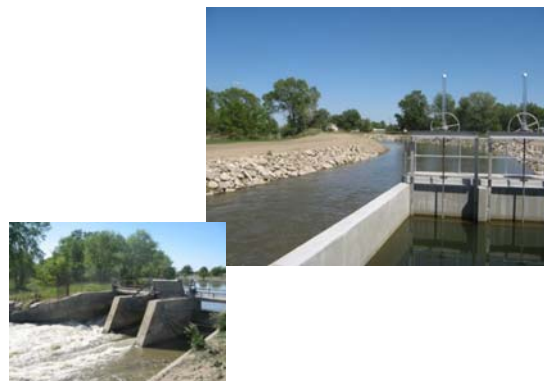
Cozad Canal, Gothenburg, NE
