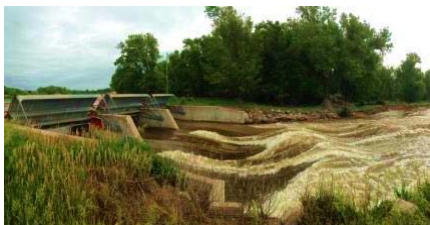
30-Mile Canal Headworks, June 2015
