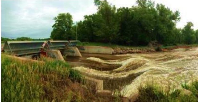
30-Mile Canal Headworks, June 2015
