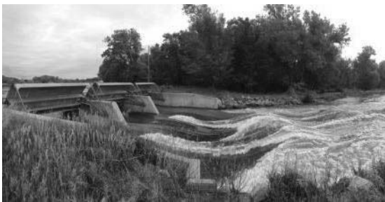
30-Mile Canal Headworks, June 2015
