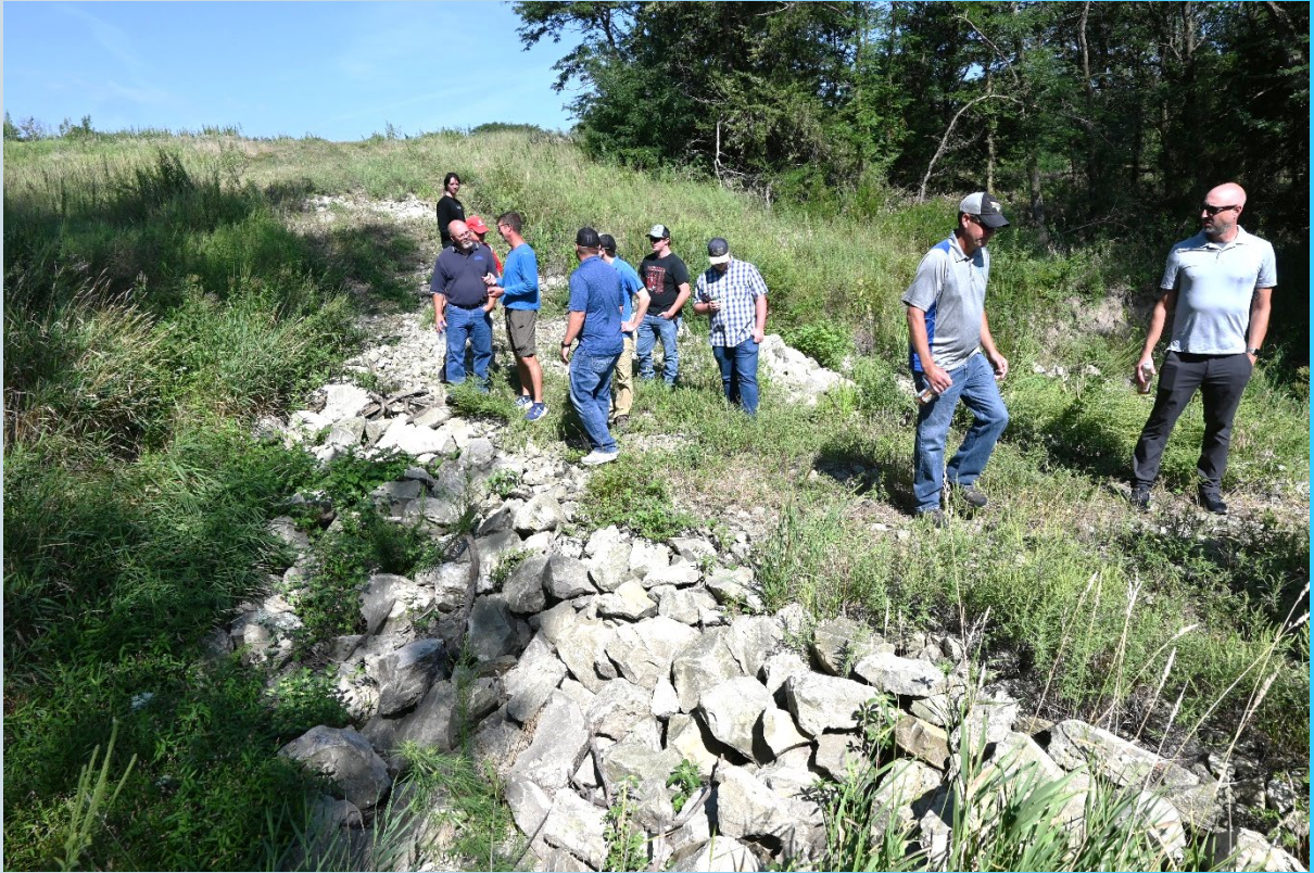
Sorensen Groundwater Recharge Weir in Southeast Kearney County
