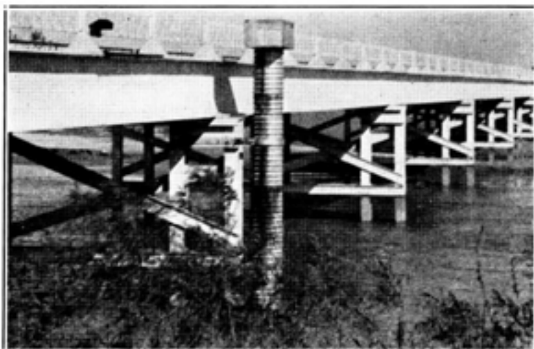
General View of Gaging Station with Recorder Shelter and Chain Gage on Bridge over Platte River near Odessa.
