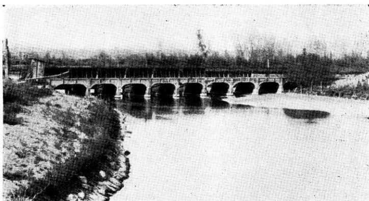
Headgates of the Tri-State Canal
