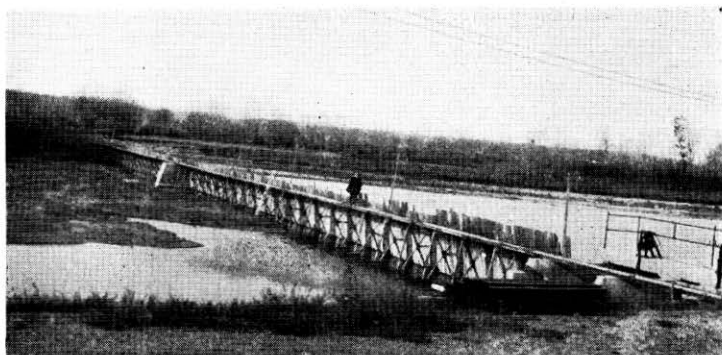
Needle Diversion Dam Tri-State Canal
