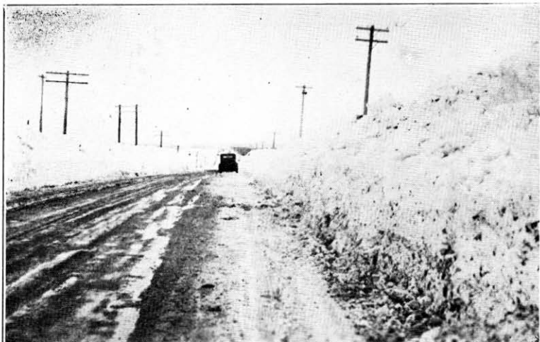
Typical view after drifts are opened.
