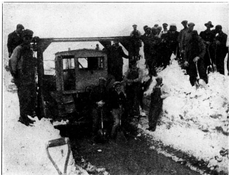
It required caterpillar tractor and plow with the help of shovelers, to open this drift.
