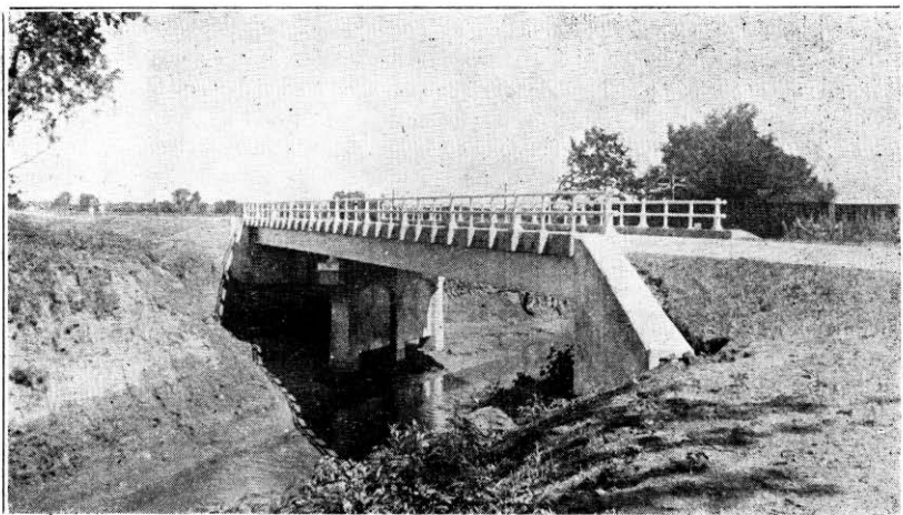
Project No. 91-A, Florence-Blair. One 76-foot and one 48-foot deck steel girder on Highway No. 36 over Mill Creek.
