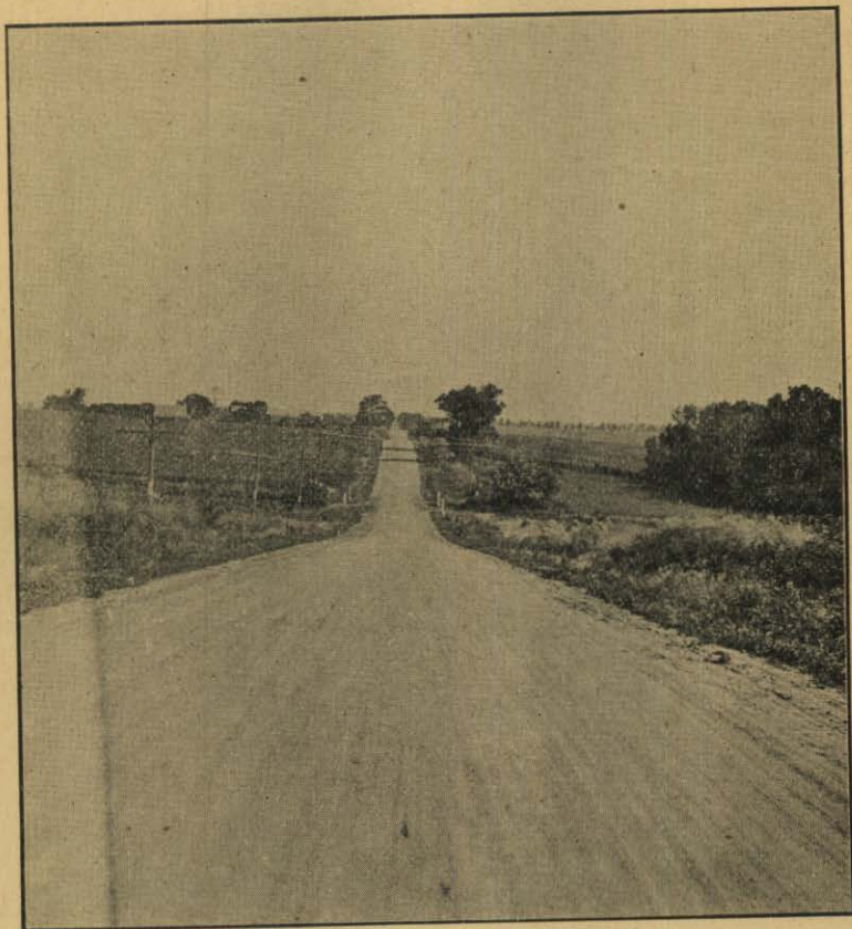
Saunders County State Highway No. 9
