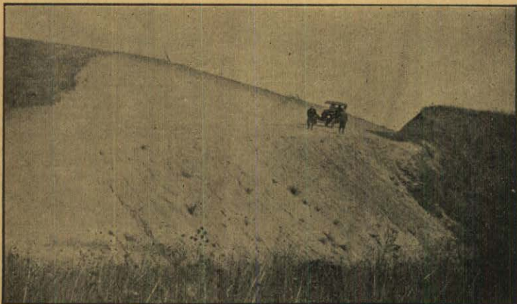
View of side hill cut and fill at the beginning of curve shown in first picture, Project 193.
