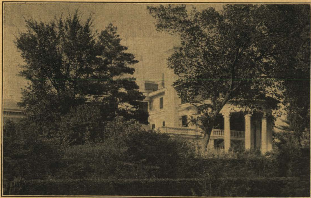
View of Arbor Lodge from Southwest
