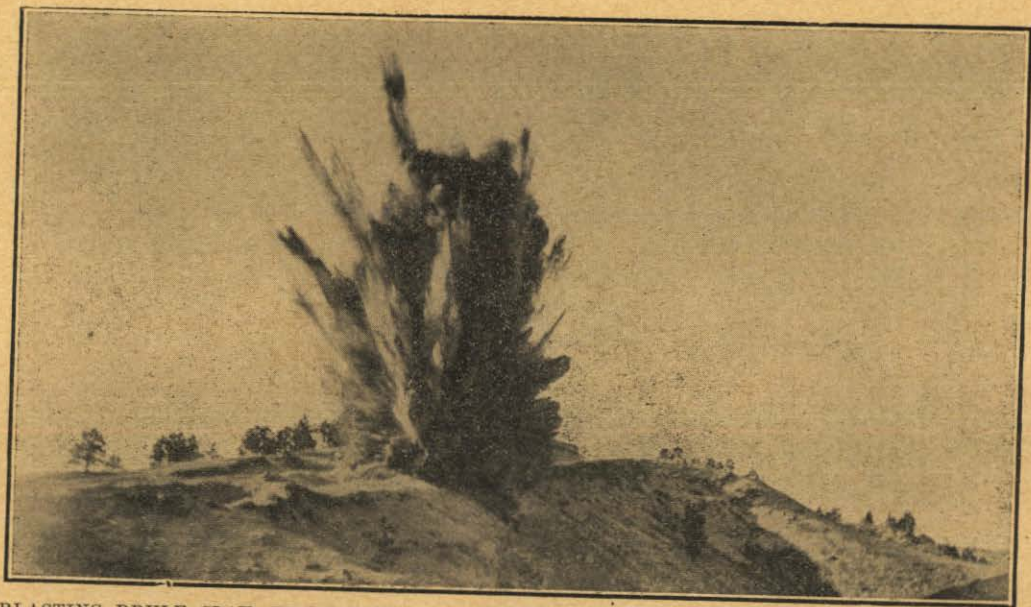
BLASTING BRULE CLAY, PROJECT NO. 66, VALENTINE-SPARKS FEDERAL AND STATE AID ROAD
