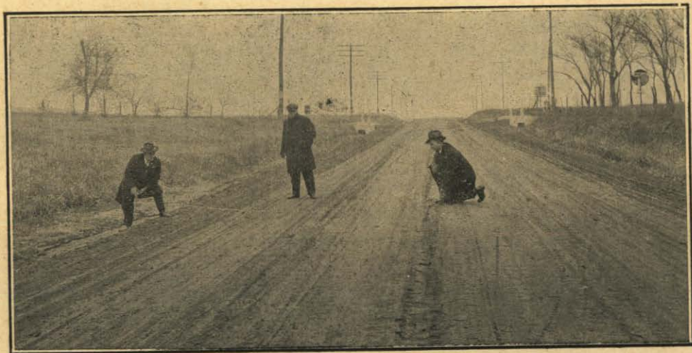
FINAL ACCEPTANCE OF A FEDERAL AND STATE AID ROAD PROJECT AFTER COMPLETION
