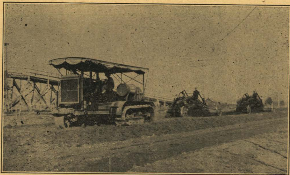
THIS HEAVY GANG MAINTENANCE CREW GRADES ROADS ON WHICH IT IS NOT NECESSARY TO MAKE HEAVY CUTS OR FILLS
