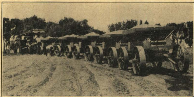
TRAILERS HAULED BY TRACTOR GRAVELLING STATE AND FEDERAL AID ROAD IN HALL COUNTY
