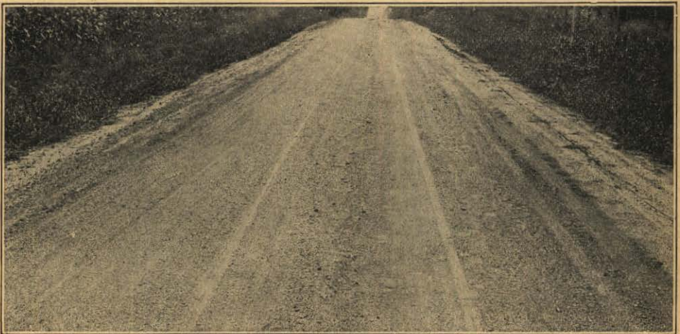
COMPLETED GRAVEL ROAD, FREMONT-CERESCO, FEDERAL AND STATE AID PROJECT NO. 27
