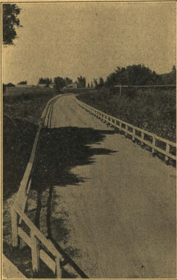
VIEW OF A COMPLETE EARTH GRADED ROAD WITH GUARD RAIL, NEAR WOOD RIVER BRIDGE
