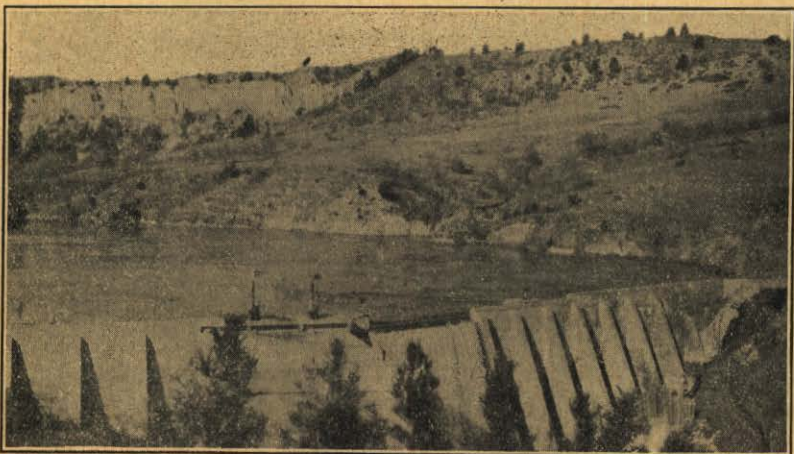
AINS WORTH POWER PLANT, PLUM CREEK
