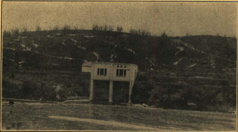
CORNELL HYDRO-ELECTRIC PLANT, VALENTINE, NEB.
