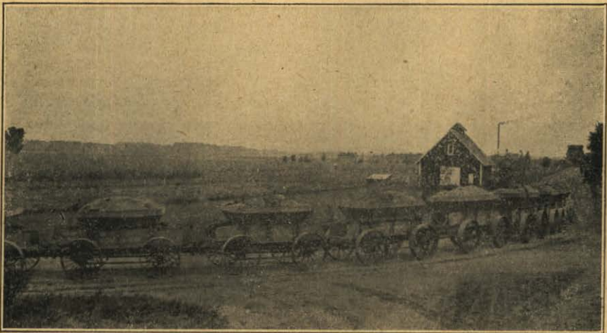
GRAVELING FREMONT-CERESCO FEDERAL AND STATE AID ROAD. PROJECT 27
