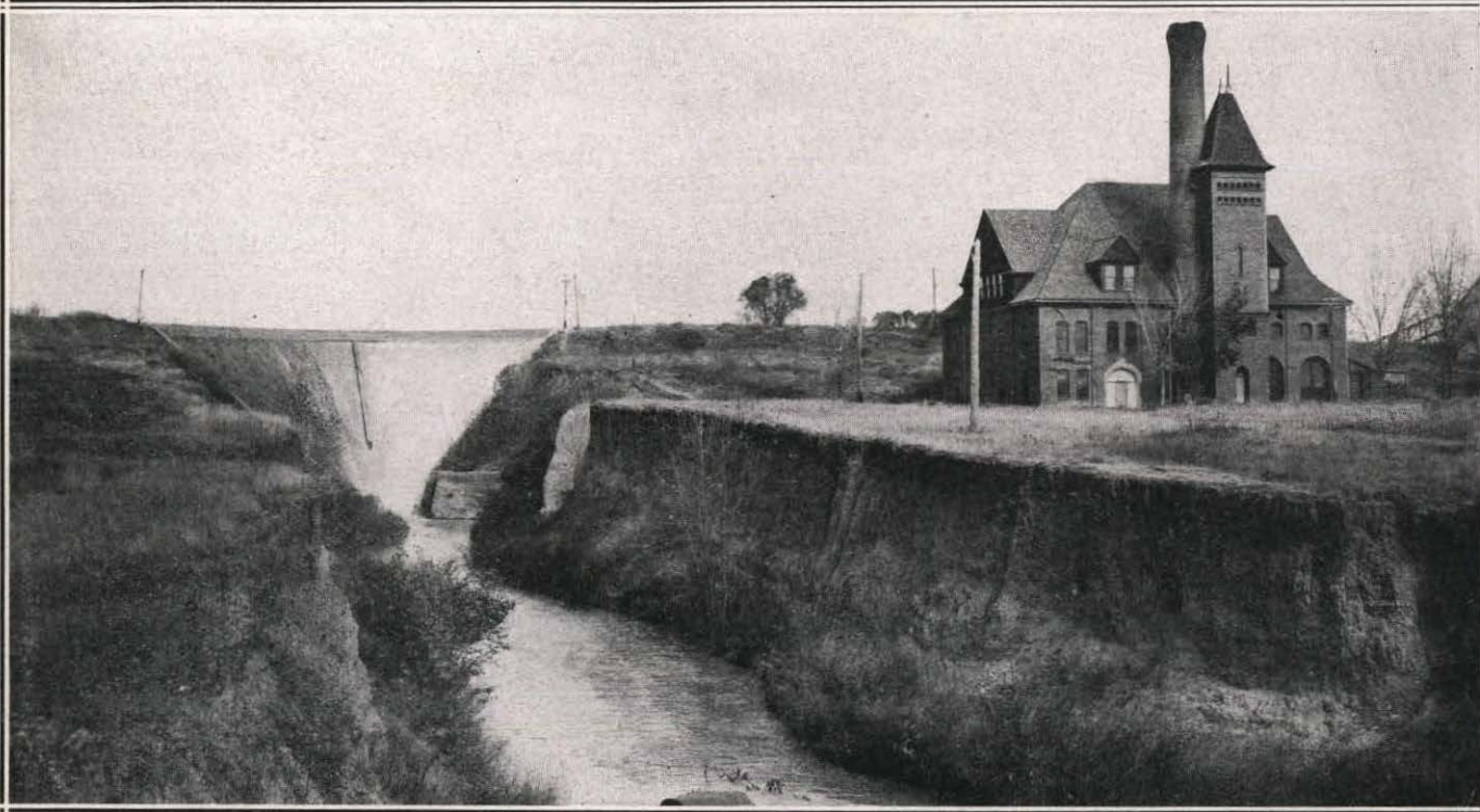
POWER HOUSE AND WASTE WEIR OF THE KEARNEY CANAL. FALL IS 60 FEET. WEIR IS 120 FEET WIDE
