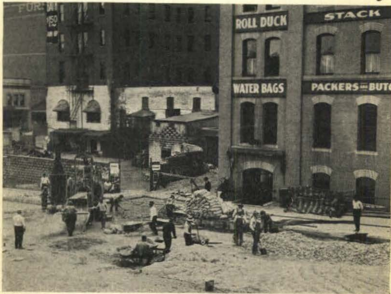
FIGURE 34 SAND USED IN STREET WORK, OMAHA
