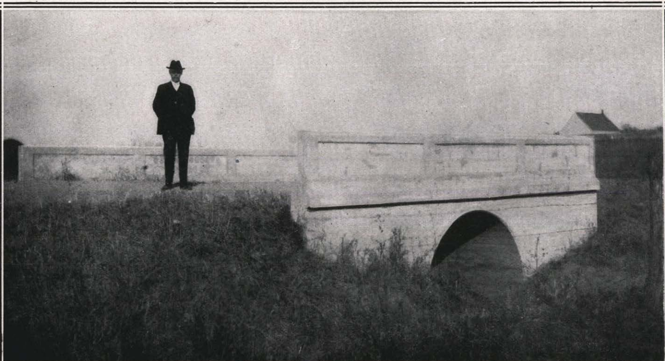
SMALL CULVERT, SEWARD COUNTY
