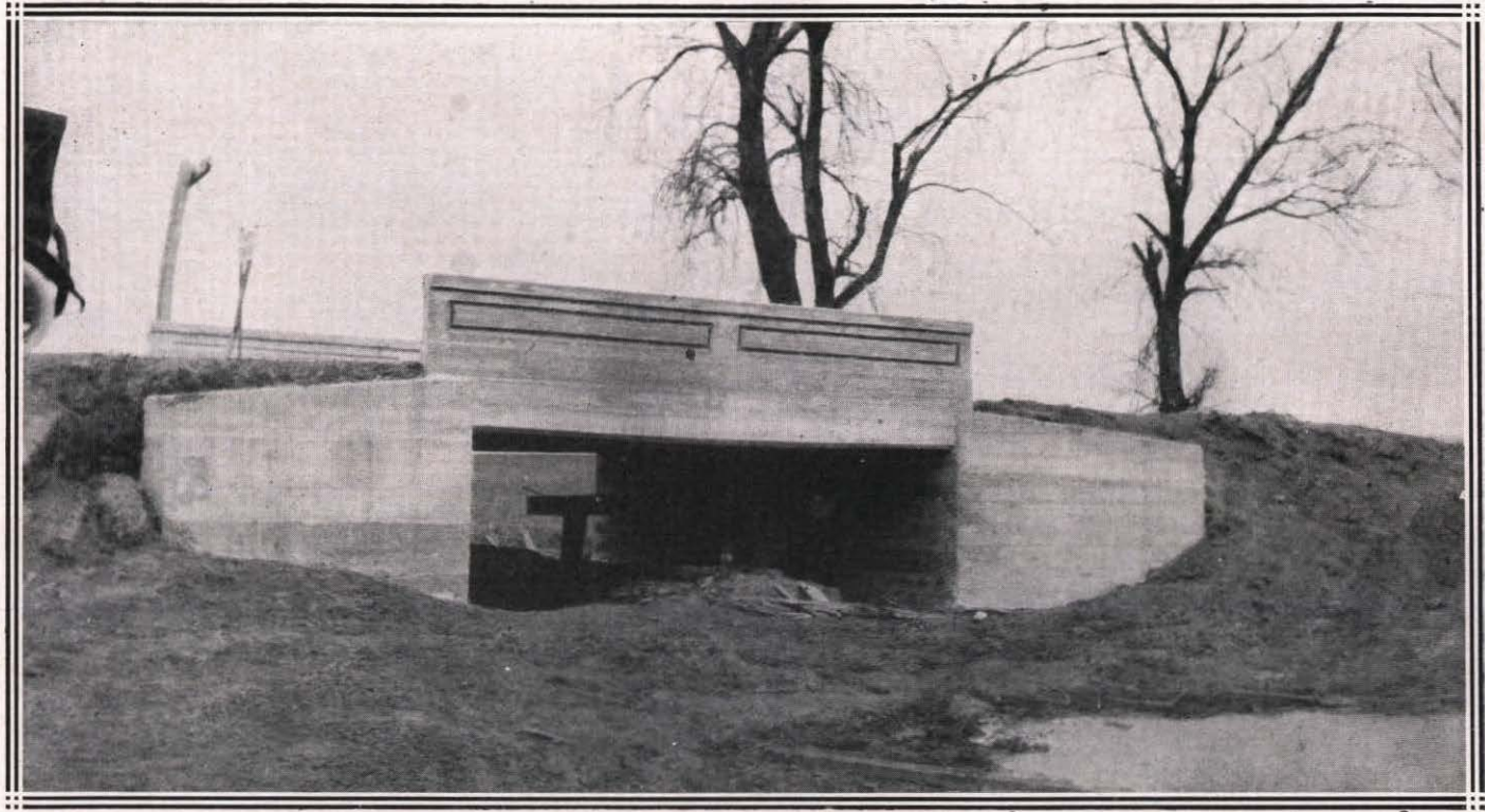
16-FT. CONCRETE SLAB, CLAY COUNTY
