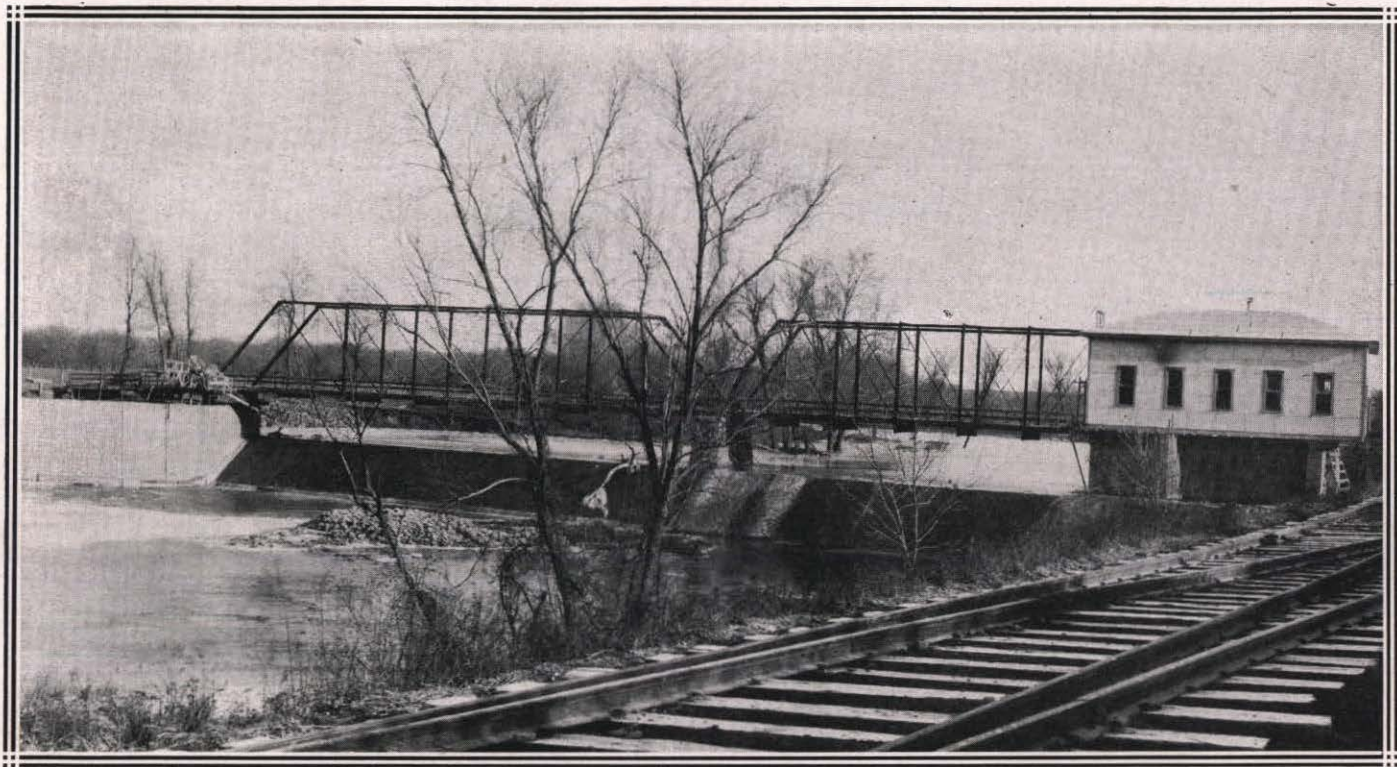
HOLMESVILLE MILL & POWER COMPANY, HOLMESVILLE, NEBRASKA
