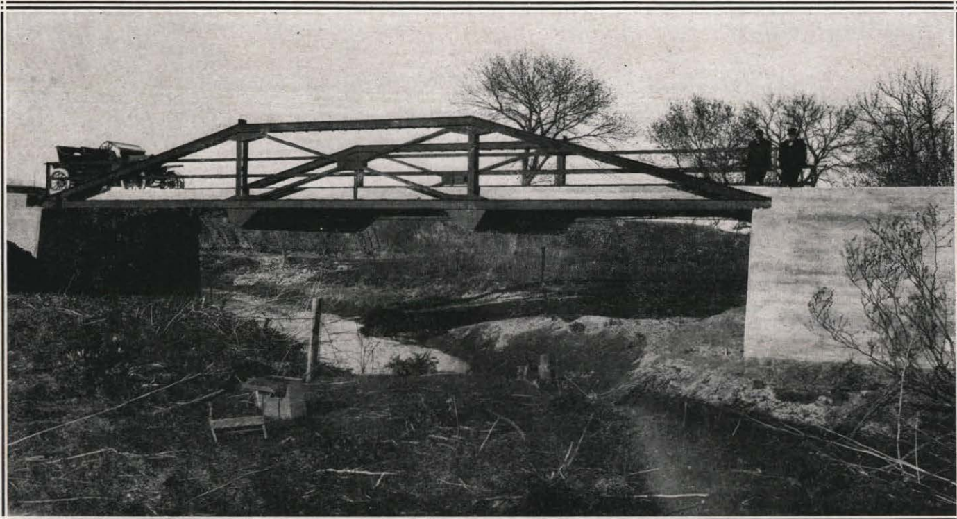
60-FT. FIFTEEN TON SPAN IN POLK COUNTY NEAR STROMSBURG
