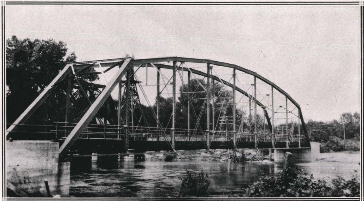
ARLINGTON STATE AID BRIDGE, ELKHORN RIVER, 1913 ONE 180-FT TRUSS
