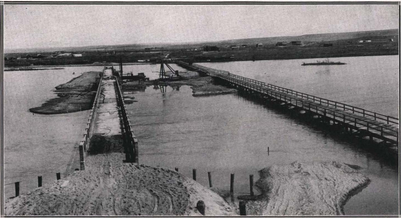
BRIDGEPORT STATE AID BRIDGE, NORTH PLATTE RIVER. BUILT 1914, TWENTY-THREE 33-FT. CONCRETE GIRDERS
