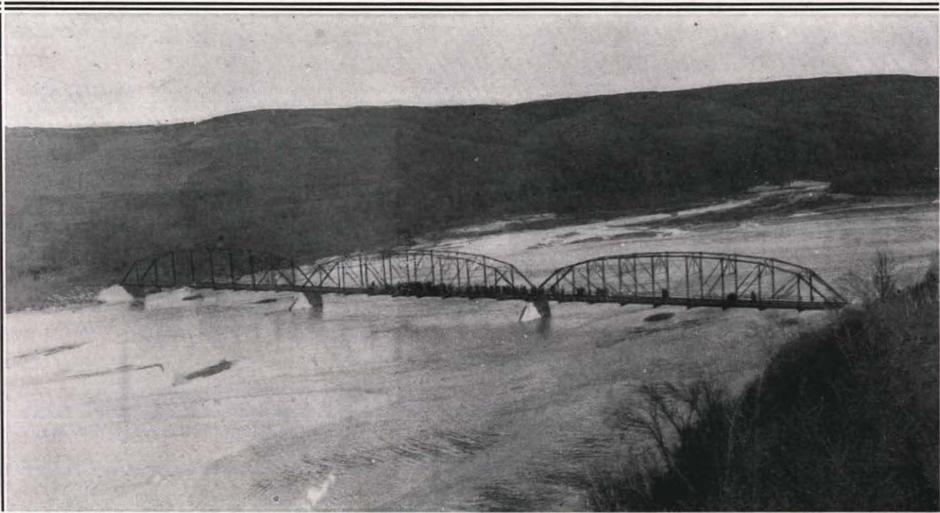
PARSHALL STATE AID BRIDGE, NIOBRARA RIVER NEAR BUTTE, 1917 THREE 170-FT. TRUSSES
