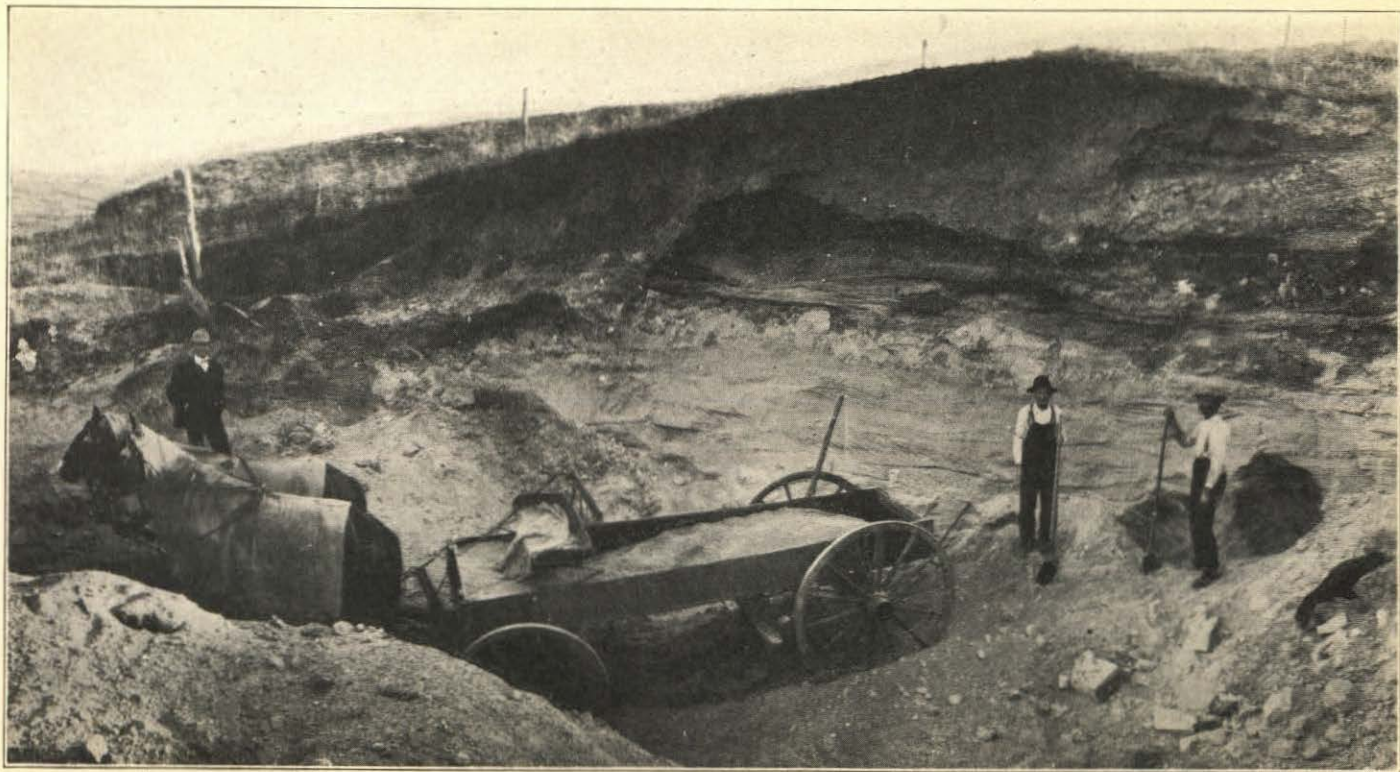
FIGURE 16 BANK SAND PIT NEAR CAMBRIDGE
