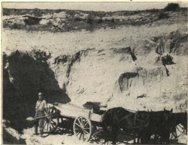
FIGURE 9 HAND SHOVELING FROM BANK PIT
