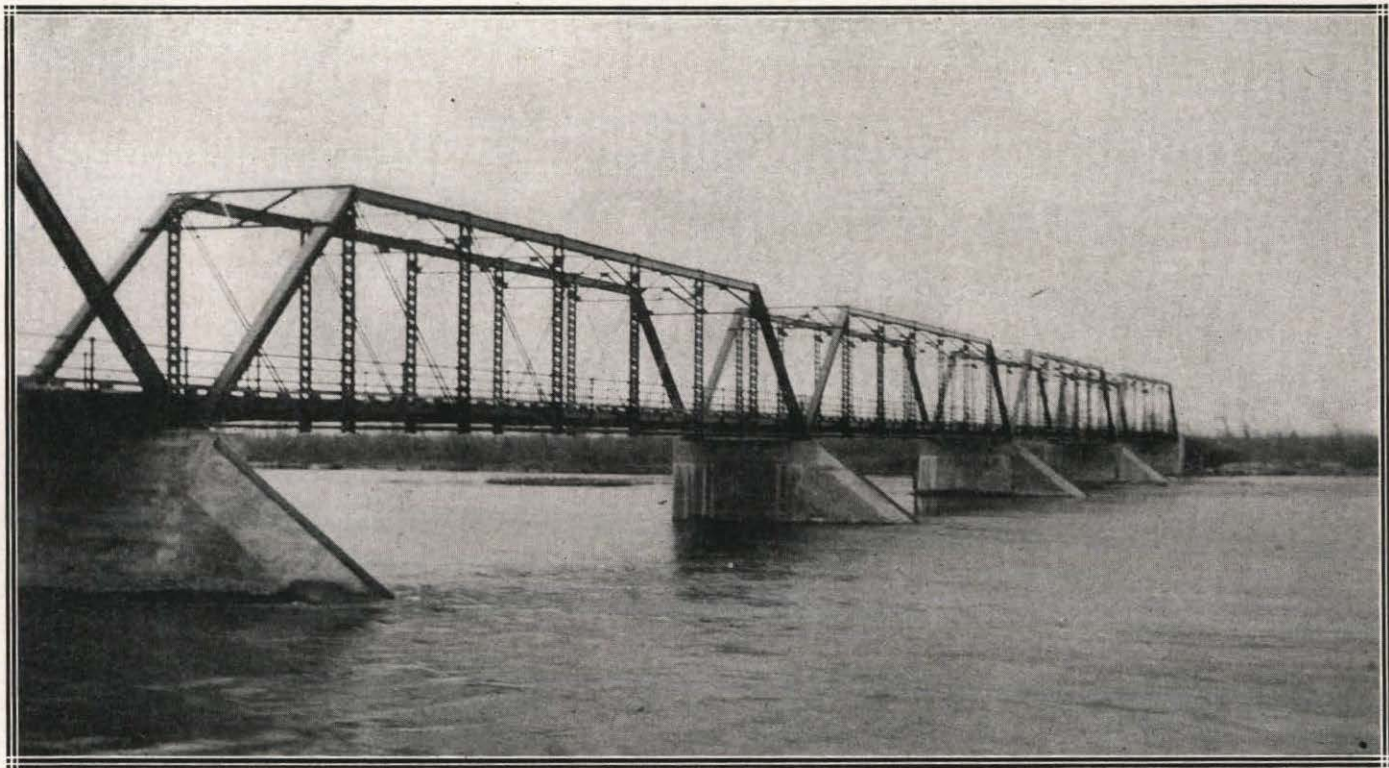
GENOA STATE AID BRIDGE, LOUP RIVER. BUILT 1913, FIVE 136.5-FT. TRUSSES
