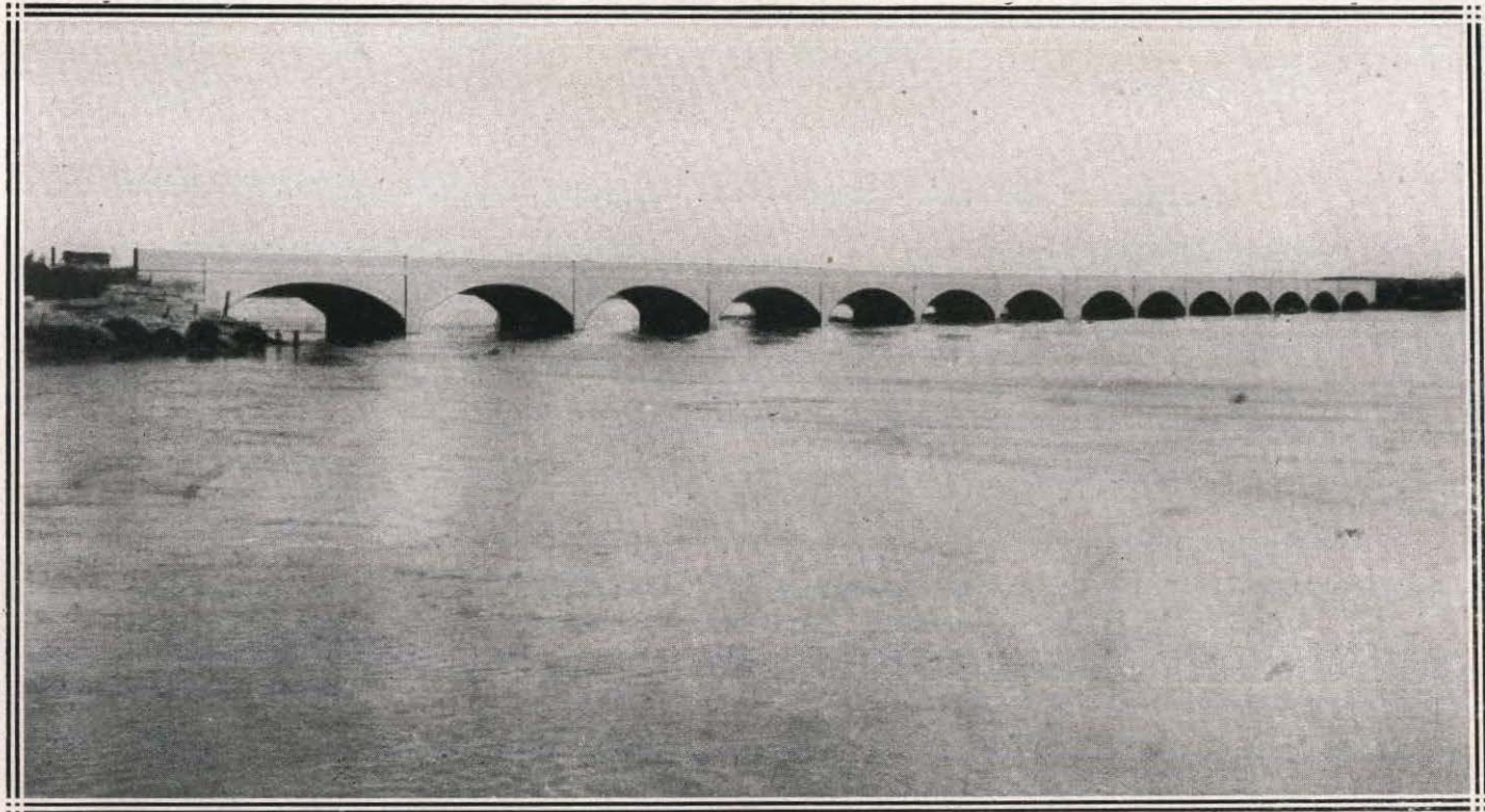
SUTHERLAND STATE AID BRIDGE, NORTH PLATTE RIVER, 1915 FOURTEEN 50-FT. CONCRETE ARCHES
