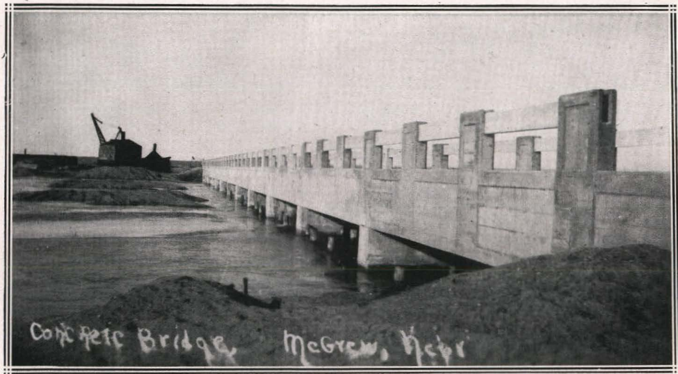
McGREW STATE AID BRIDGE, NORTH PLATTE RIVER, 1914 TWENTY-THREE 33-FT. CONCRETE GIRDERS
