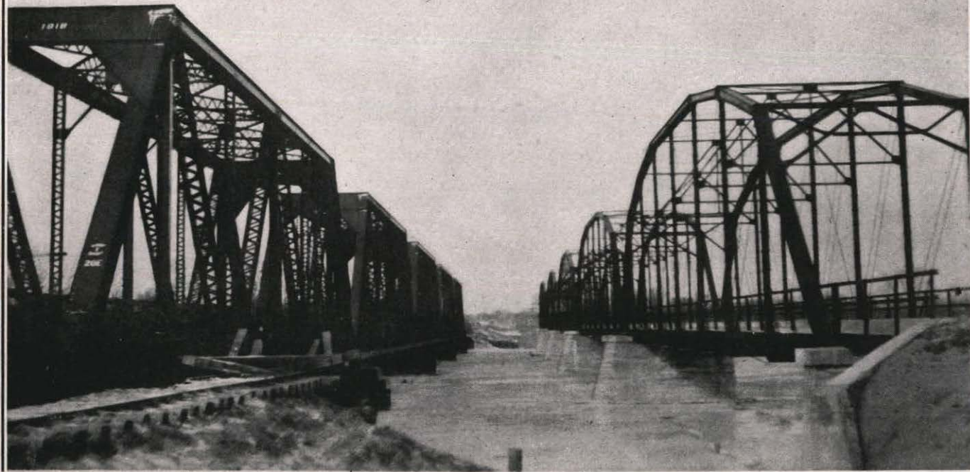
ST. PAUL STATE AID BRIDGE, LOUP RIVER, 1916 FIVE 145-FT. TRUSSES, ONE 20-FT. APPROACH
