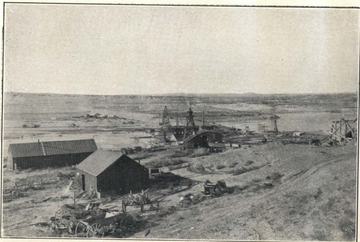
DIVERSION DAM INTERSTATE CANAL, DEC. 1908.
