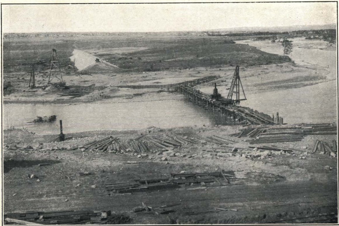
DIVERSION DAM INTERSTATE CANAL, AUG. 1907
