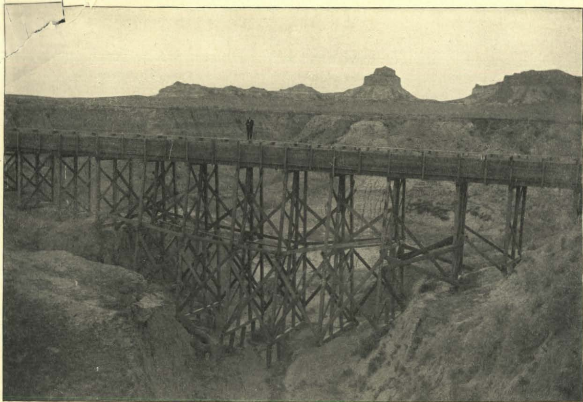
FLUME ON GERING CANAL.
