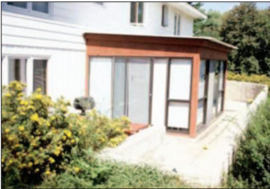
Figure 5F-2. Typical residential floodwall
