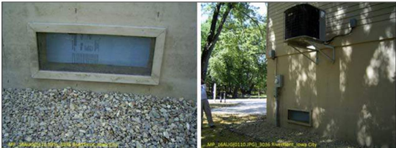
Figure 5E-14. A house where flood openings have been covered by insulation and drywall
