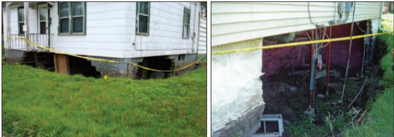
Figure 5D-14. This house’s foundation walls were not able to withstand the forces applied during or after the flood. Rebar would need to be added to help with reinforcement of the CMU foundation.
