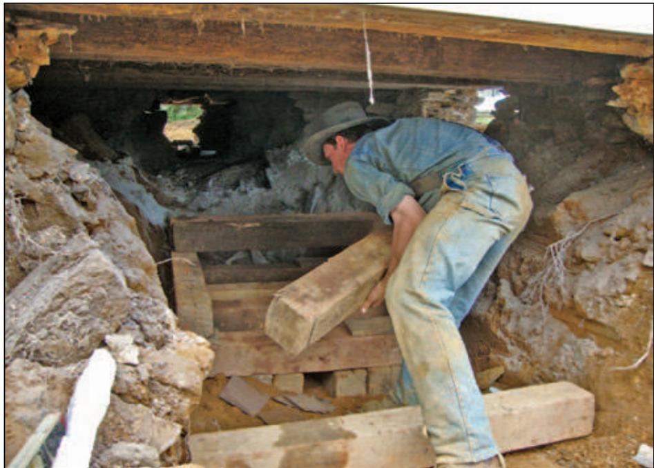
**Install Beams:** Lifting and lateral beams are placed beneath the structure at all critical lift points and support cribbing is added as the structure is separated from its old foundation (see Figure 5R-6).
