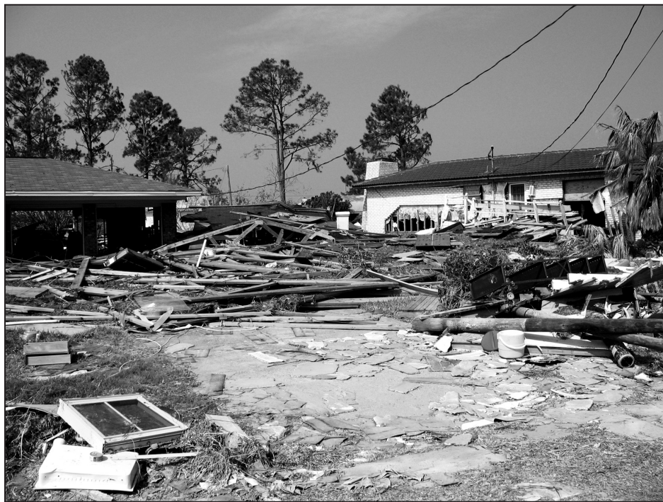
Figure 18. Homes in AE zone devastated by wave forces and debris
