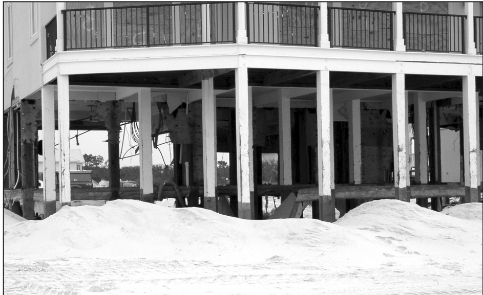
Figure 3. Successful breakaway wall performance
