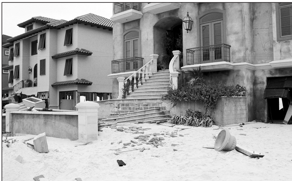
Figure 4. Non-compliant stairs
