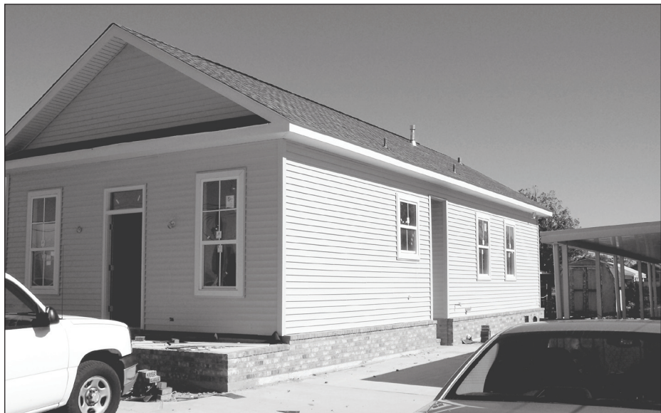
Figure 7-21. Typical mitigation reconstruction project.
