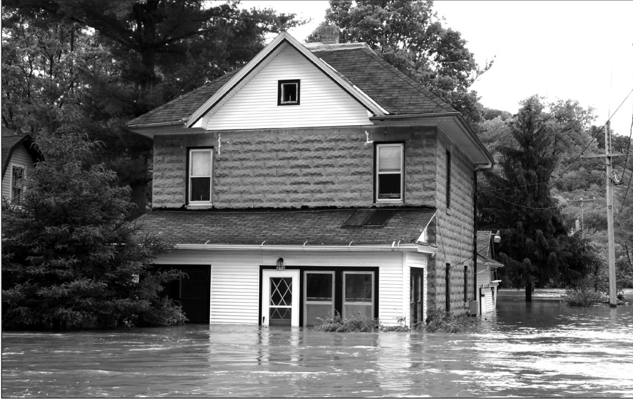
Figure 2-4. This home in Wisconsin was inundated by riverine flooding.
