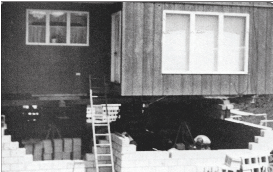
Figure 7-4. After the home is raised into place, the foundation is completed.
