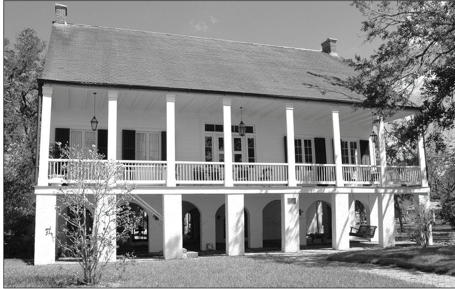
Figure 5-3. With attention to detail and planning, homeowners have created attractive retrofitted homes.
