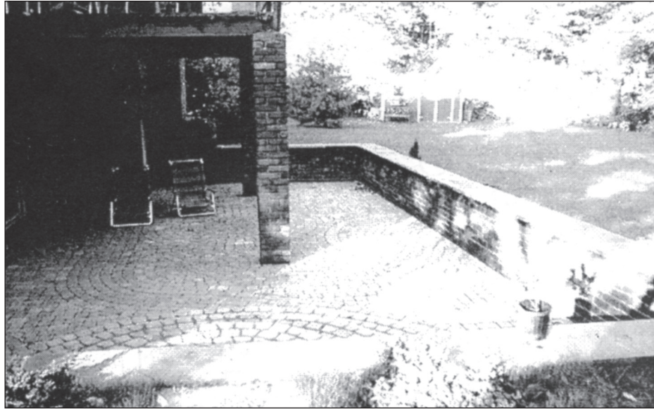
Figure 3-12. A home protected by a floodwall designed as a landscaping feature.
