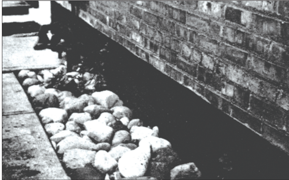
Figure 7-7. A 12-inch high asphalt coating was added to this brick wall.
