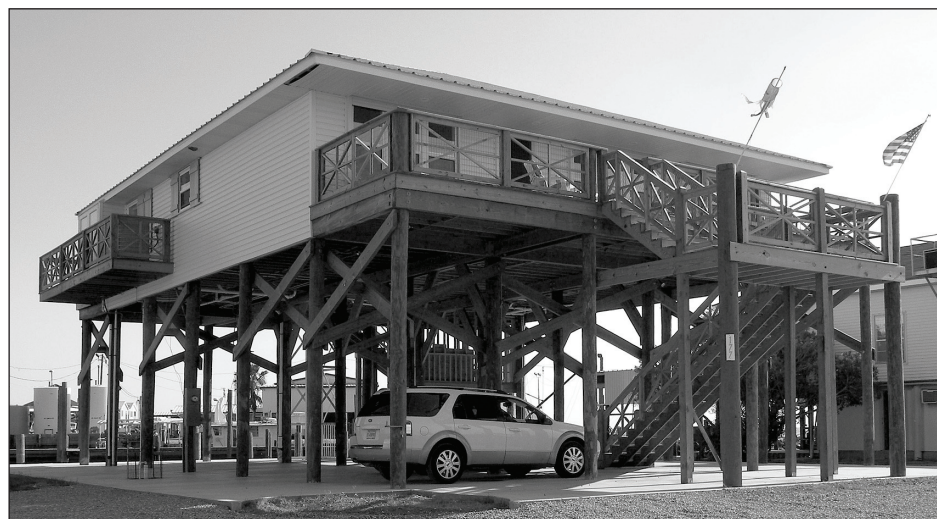
Figure 3-5. This coastal home was elevated on piles so that it is less vulnerable to damage from coastal flooding.
