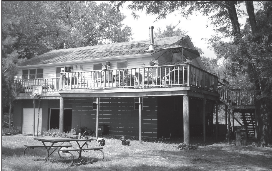
Figure 5-2. This home in Cedar Falls, Iowa, was elevated one full story. The garage and storage area are at the home's original elevation.
