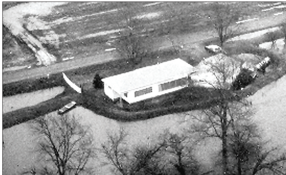
Figure 3-11. A home protected by a levee, which holds back the floodwaters shown in the lower half of the photograph. Note that the levee ties in to high ground created by the road embankment.
