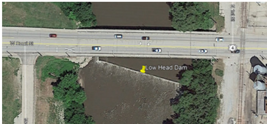
Top: Dangerous low head dam in the Big Blue River under the Court Street Bridge in Beatrice. Photo by NeDNR Staff.
