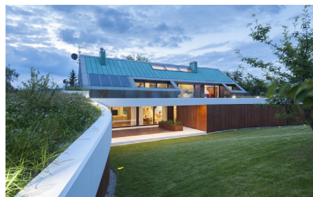
Example of grading resulting in a positive flow toward the house. Copyright 2015, Mobius.
