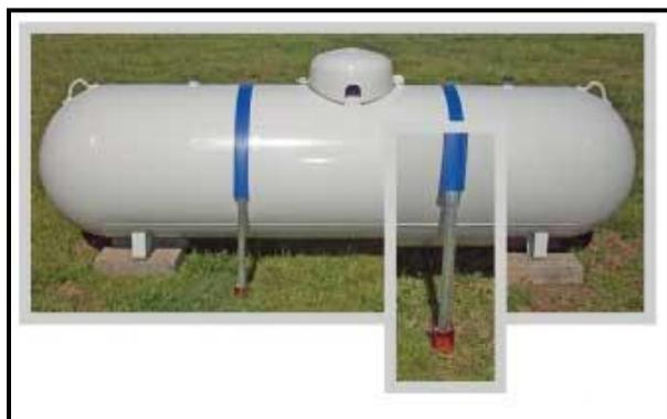
Figure 5. Typical anchoring system (photo used with permission from Tarantin Industries)
