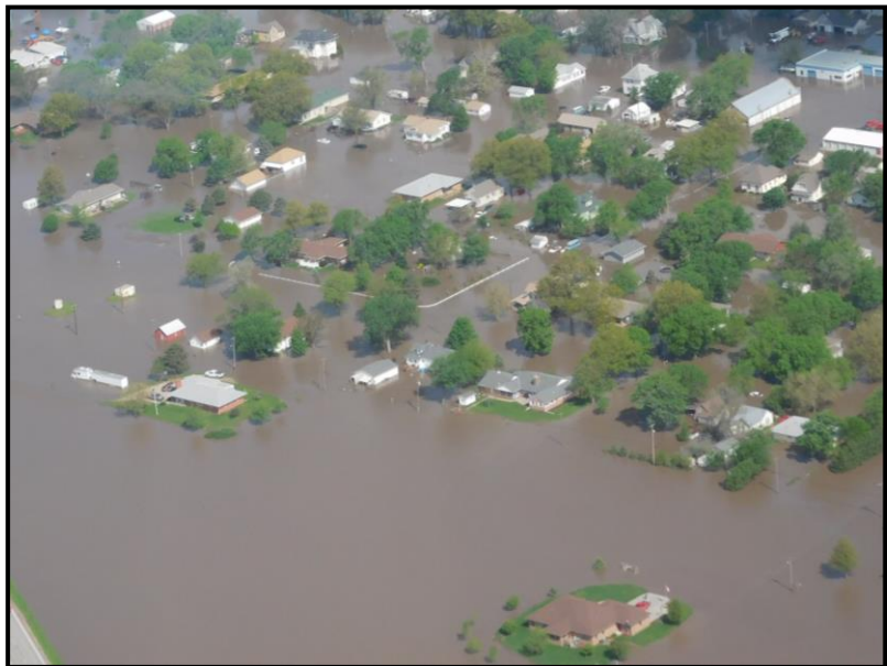
Figure 5. Fill in the floodplain in DeWitt pushes water on neighboring properties
