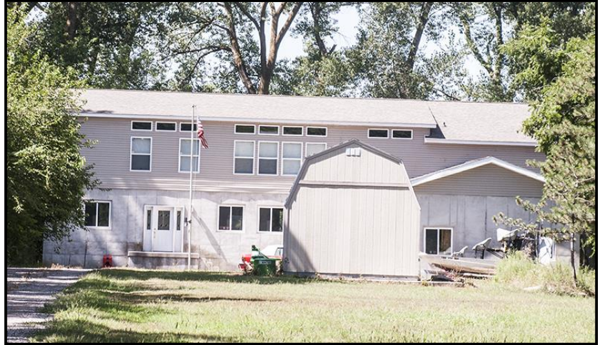
Figure 3. Home along the Platte River with a converted crawlspace
