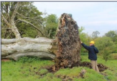
Uprooted trees can remove a significant portion of a dam.
