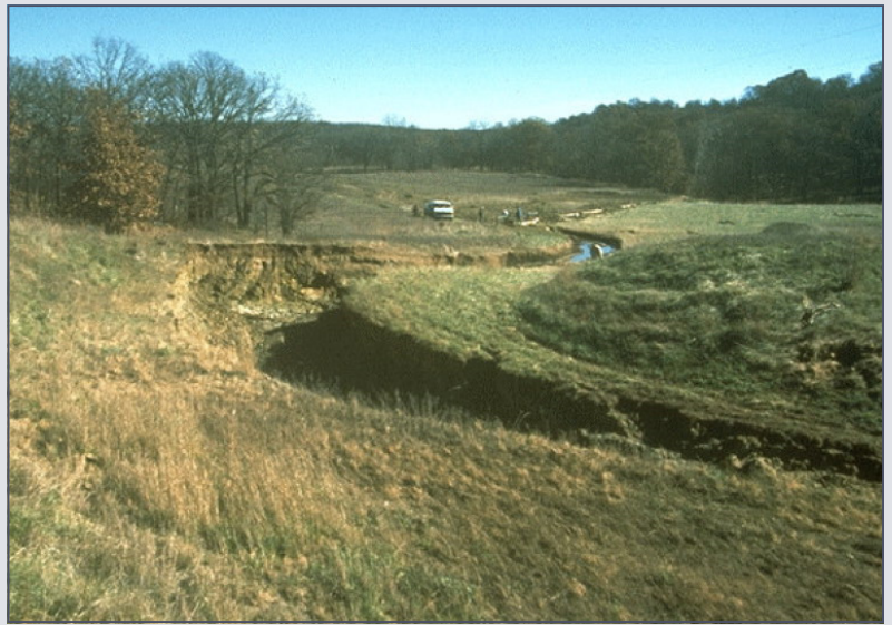
Vehicle paths in the auxiliary spillway led to failure of this dam in Kansas. Vehicle ruts and cattle trails in earthen spillways must be repaired and reseeded to prevent erosion. (Photo source: Darrel Temple)
