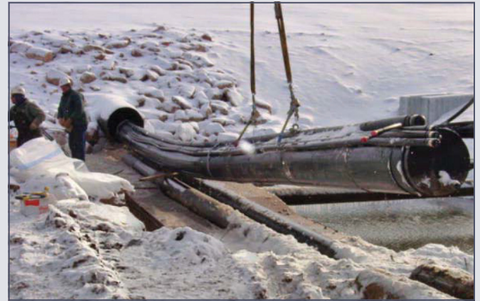
Rusty corrugated metal pipes can be sliplined with pressure-tight, solid-wall, HDPE pipe. Grout is injected into the space between the old and new pipes. (Photo source: FEMA)
