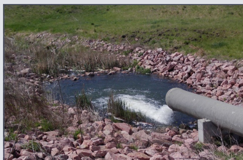
A well-designed plunge pool (left, right) or stilling basin (center) can prevent erosion at the outlet of spillway pipes.
