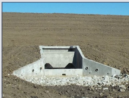
A well-designed plunge pool (left, right) or stilling basin (center) can prevent erosion at the outlet of spillway pipes.
