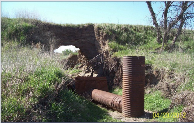
Corrosion of the corrugated metal principal spillway pipe led to this dam failure in Adams County.
