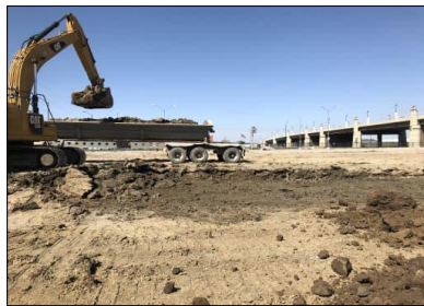
Excavation and disposal of contaminated soil
