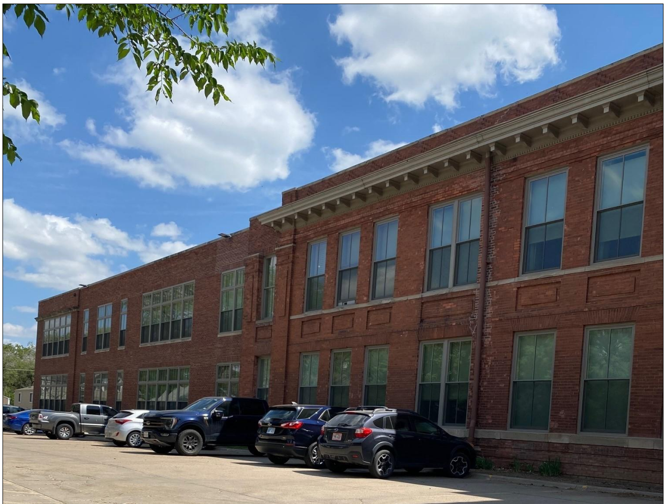
Pictured Above: Single-Family and Multi-Family Residential Projects. Top Row: New Air Conditioning Condenser (top-left), Window Replacements (top-center), New Photovoltaic System (top-right). Bottom Row: Hayward Place Condominiums - $367 thousand window replacement project.
