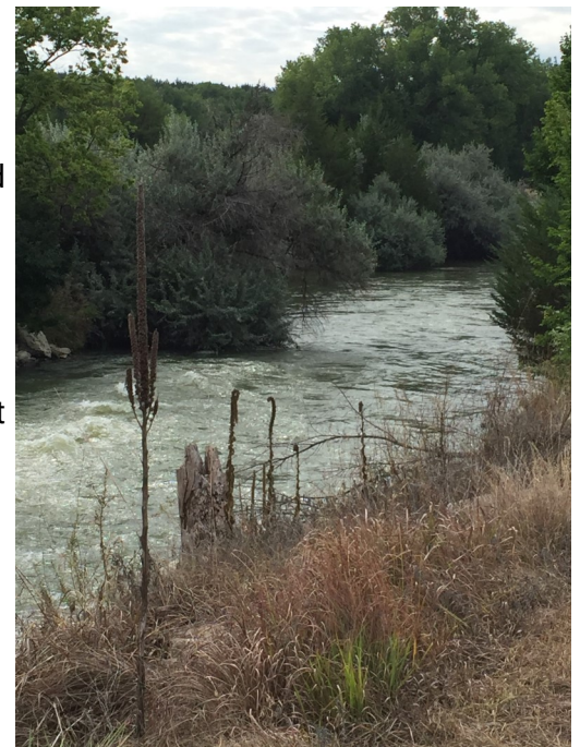
Outlet at Harlan County Dam
