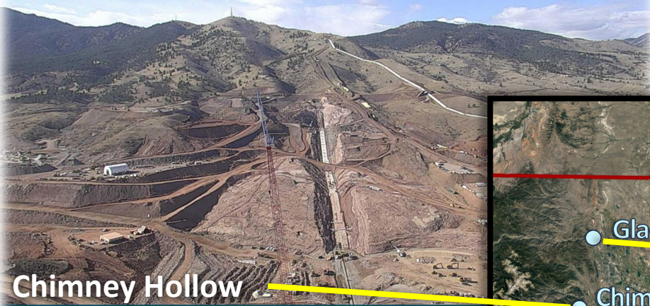
Chimney Hollow Reservoir Project
